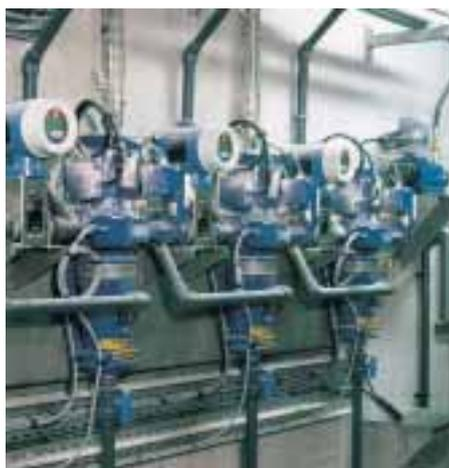
Three MV1200F4 pumps with cast iron bodies from a set of 7 waste water treatment plant polymer dosing pumps. These pumps ensure injection proportional to a sludge flow into a dewatering unit with a centrifugal decanter.
